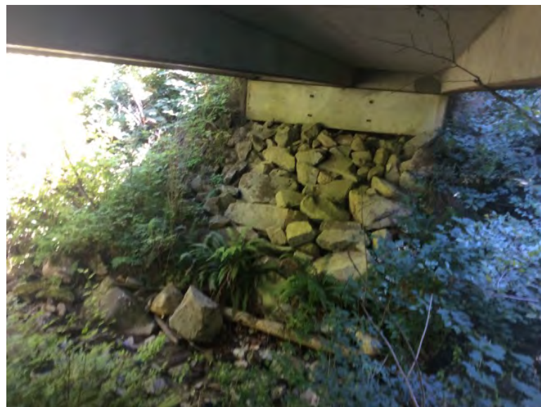
Left Bank Abutment when facing downstream
