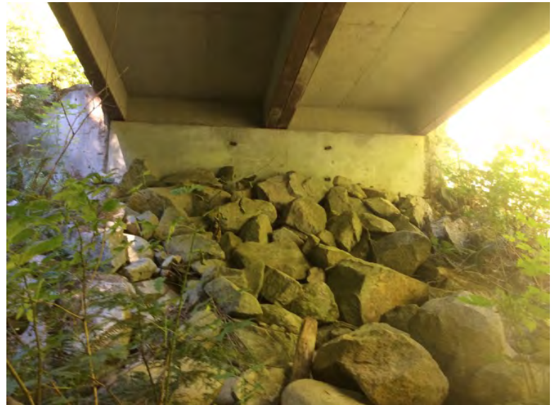
Right Bank Abutment when facing downstream
