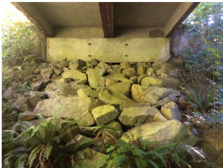
Left Bank Abutment when facing downstream
