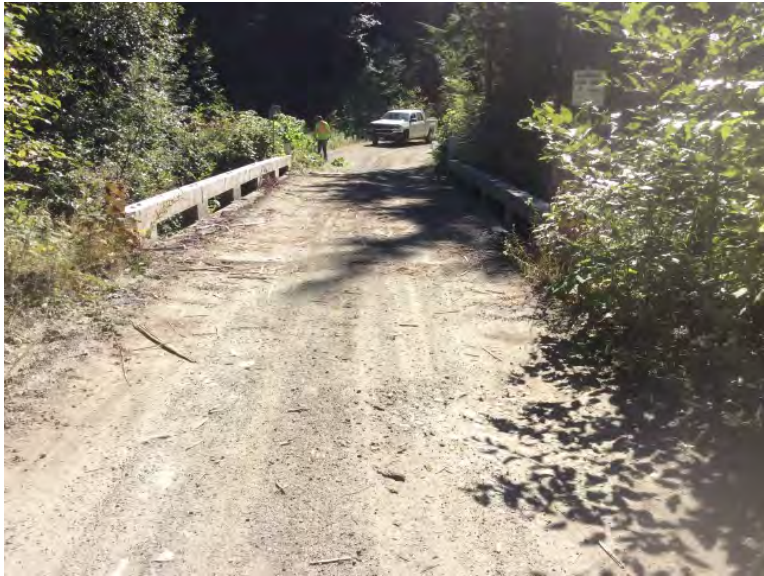
Approach from Right Bank when facing downstream
