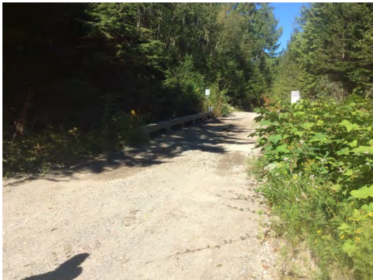
Approach from Left Bank when facing downstream
